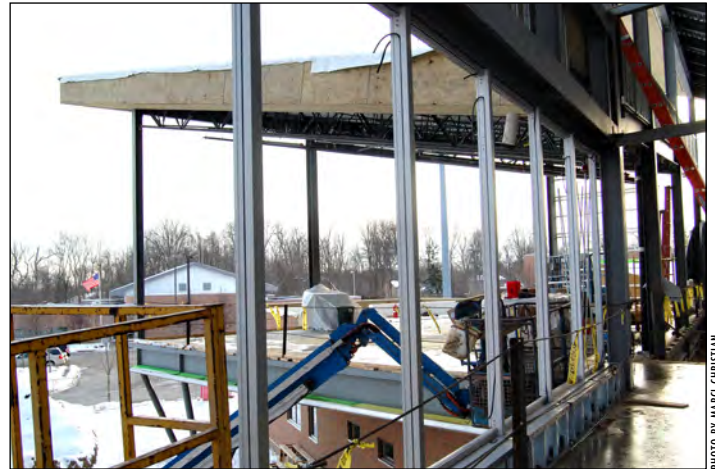
B & A Steel Co., Inc., Chesterfield, erected the structural steel for this angular building's hybrid block and steel frame structure.
