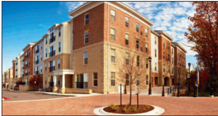
Courtyards Housing Campus, U of M Ann Arbor CM/GC: T.H. Marsh Construction Co. Architect: Neumann/Smith Associates
