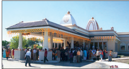
Hindu Temple of Canton Canton CM/GC: Rand Construction Engineering, Inc. Architect: Lindhout Associates
